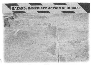
**Damage – Uneven Edges**Uneven edges and the attempted repair need to be ground down and filled with a flexible epoxy.
