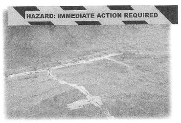
**Damage - Uneven Edges**Uneven edges and the attempted repair need to be ground down and filled with a flexible epoxy.
